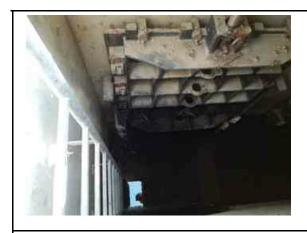
Inspect ID: 2020-0062 Title: 2604000003\_CELRC\_2020\_A\_2020-0062\_2\_20200512T155947.jpg Rated Item: 10. Sluice/ Slide Gates Caption: Acceptable - GN-8: Able to see GN-8a and GN-8b closed but can't see GN-8c. GN-8a and GN-8b closed fully. Operated GN-8c up and down.
