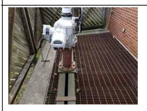
Inspect ID: 2021-0006 Title: 2604000010\_CELRC\_2021\_A\_2021-0006\_1\_20210621T150052.jpg Rated Item: 18. Sluice/ Slide Gates Caption: Acceptable - PS-SH: Sluice gate not initially working, it was over-torqued in the open position. It was repaired. Inspection showed that sluice gate closes as long as gate is left open less than 95%. Issue has been resolved. Recommend adding label to warn operators not to over-open gate.
