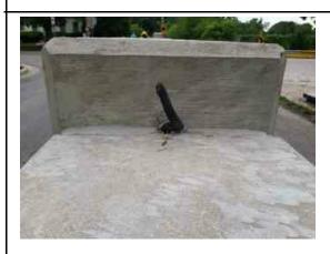
Inspect ID: 2021-0009 Title: 2604000010\_CELRC\_2021\_A\_2021-0009\_3\_20210624T145137.jpg Rated Item: 7. Monolith Joints Caption: Minimally Acceptable - Exposed filler material. Typical along wall. Reseal.
