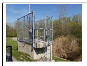
Inspect ID: 2021-0004 Title: 2604000006\_CELRC\_2021\_A\_2021-0004\_2\_20210427T143733.jpg Rated Item: 10. Sluice/ Slide Gates Caption: Acceptable - GR-2: The sluice gate opened and closed with little to no resistance. The gate stem appears to be oiled regularly. The gate was open on arrival and we left it open when we left.
