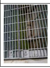
Inspect ID: 2021-0145 Title: 2604000008\_CELRC\_2021\_A\_2021-0145\_1\_20210623T162942.jpg Rated Item: 10. Sluice/ Slide Gates Caption: Minimally Acceptable - HA-16: The sluice gate opens and close fully but there is a lot of resistance. Recommend greasing. There is a lot of sediment in the gate pit. Recommend cleaning. Mild corrosion on the railing. The gate was closed when we arrived we left it closed when we left.
