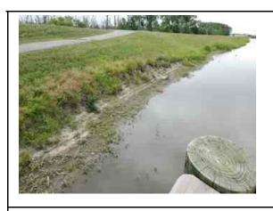
Inspect ID: 2021-0632 Title: 2604000008\_CELRC\_2021\_A\_2021-0632\_2\_20210623T191847.jpg Rated Item: 6. Erosion/ Bank Caving Caption: Minimally Acceptable - Typical erosion along riverside toe. Armor.
