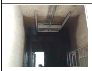
**Inspect ID:** 2021-0105 **Title:** \_1\_20210623T150005.jpg **Rated Item:** 10. Sluice/ Slide Gates **Caption:** Acceptable - HA-13: The sluice gate is in good condition. It opened and closed completely. It was opened when we arrived we left it open when we left.
