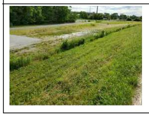
Inspect ID: 2021-0108 Title: 2604000008\_CELRC\_2021\_A\_2021-0108\_2\_20210623T134922.jpg Rated Item: 1. Unwanted Vegetation Growth Caption: Minimally Acceptable - Tall veg from lack of mowing around stakes on landside. Remove stakes and mow.
