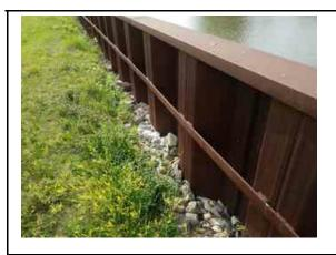
Inspect ID: 2021-0197 Title: 2604000008\_CELRC\_2021\_A\_2021-0197\_2\_20210624T131220.jpg Rated Item: 6. Foundation of Concrete Structures Caption: Minimally Acceptable - Settlement again sheet pile. Fill to drain away from the wall.
