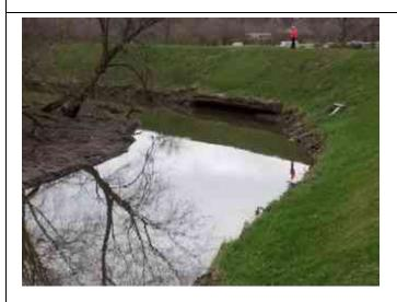
Inspect ID: 2022-0081 Title: 2604000010\_CELRC\_2022\_A\_2022-0081\_2\_20220413T185703.jpg Rated Item: 13. Revetments other than Riprap Caption: Minimally Acceptable - Retaining wall on riverside toe is tilting.
