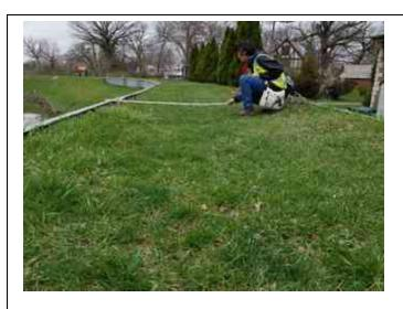
Inspect ID: 2022-0061 Title: 2604000010\_CELRC\_2022\_A\_0061\_1\_20220413T184249.jpg Rated Item: 5. Tilting, Sliding or Settlement of Concrete Structures Caption: Minimally Acceptable - Settling of soil within bin wall, likely due to expanding walls mentioned in 2022-045. Fill to maintain top of levee elevation as necessary.
