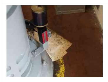
Inspect ID: 2022-0016 Title: 2604000010\_CELRC\_2022\_A\_0016\_1\_20220411T152819.jpg Rated Item: 7. Pumps Caption: Minimally Acceptable - PS-FA: Pump SWP1 showing some signs of leaking around exterior base of pump.
