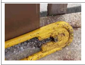
Inspect ID: 2022-0004 Title: 2604000010\_CELRC\_2022\_A\_0004\_1\_20220411T150933.jpg Rated Item: 5. Plant Building Caption: Minimally Acceptable - PS-SH: Crack along building stairway.
