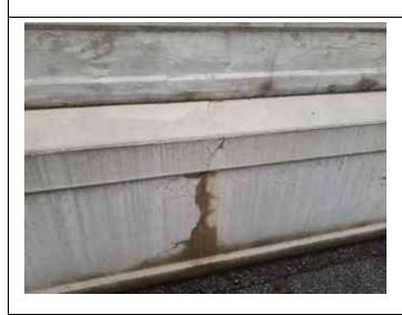
Inspect ID: 2022-0093 Title: 2604000010\_CELRC\_2022\_A\_0093\_1\_20220413T191845.jpg Rated Item: 4. Concrete Surfaces Caption: Minimally Acceptable - Crack on landside of floodwall.
