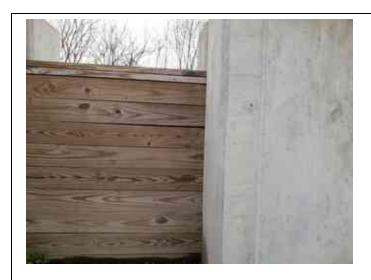
Inspect ID: 2022-0083 Title: 2604000010\_CELRC\_2022\_A\_0083\_1\_20220413T190155.jpg Rated Item: 3. Closure Structures (Stop Log Closures and Gates) (A or U only) Caption: Acceptable - South closure. Stop logs are warping and would leak when loaded.
