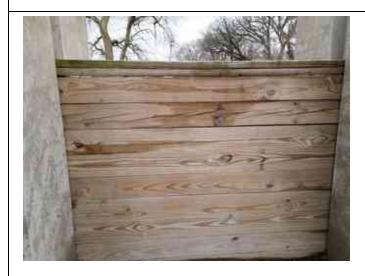
Inspect ID: 2022-0089 Title: 2604000010\_CELRC\_2022\_A\_0089\_1\_20220413T191225.jpg Rated Item: 3. Closure Structures (Stop Log Closures and Gates) (A or U only) Caption: Acceptable - North closure. Stop logs are warping and would leak when loaded.
