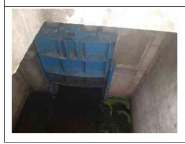
Inspect ID: 2022-0014 Title: 260400003\_CELRC\_2022\_A\_0014\_1\_20220606T161759.jpg Rated Item: 10. Sluice/ Slide Gates Caption: Acceptable - Gate 950: Completely opened, no sediment.
