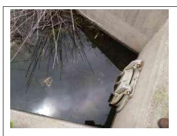
Inspect ID: 2022-0062 Title: 2604000003\_CELRC\_2022\_A\_0062\_1\_20220607T172716.jpg Rated Item: 11. Flap Gates/ Flap Valves/ Pinch Valves Caption: Minimally Acceptable - GN-13: Flap gate stuck open. Sandbags in outlet.
