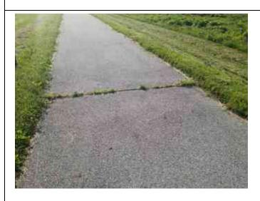
Inspect ID: 2022-0502 Title: 2604000003\_CELRC\_2022\_A\_0502\_1\_20220610T131442.jpg Rated Item: 9. Cracking Caption: Minimally Acceptable - Wide crack in the asphalt on the crest with vegetation growing in it.
