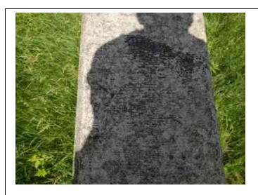
Inspect ID: 2022-0436 Title: 2604000003\_CELRC\_2022\_A\_0436\_1\_20220609T190840.jpg Rated Item: 4. Concrete Surfaces Caption: Minimally Acceptable - Crack on top of flood wall that is seen on both side faces. Penetrates 1 ft from top.
