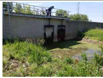
Inspect ID: 2022-0116 Title: 2604000003\_CELRC\_2022\_A\_0116\_1\_20220609T160222.jpg Rated Item: 10. Sluice/ Slide Gates Caption: Minimally Acceptable - GN-10a: Gate closed completely, when closing gate was skipping or jumping.
