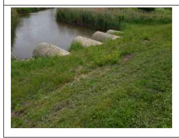
Inspect ID: 2022-0232 Title: 2604000003\_CELRC\_2022\_A\_0232\_1\_20220607T171116.jpg Rated Item: 2. Sod Cover Caption: Minimally Acceptable - Poor sod cover above culverts on riverside.
