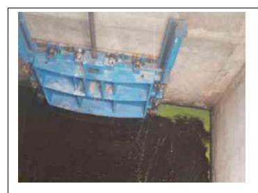
Inspect ID: 2022-0011 Title: 2604000003\_CELRC\_2022\_A\_0011\_1\_20220606T161234.jpg Rated Item: 10. Sluice/ Slide Gates Caption: Acceptable - Gate 950: Gate closed completely.
