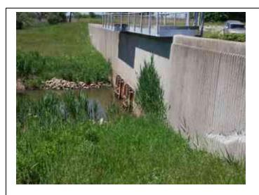
Inspect ID: 2022-0113 Title: 2604000003\_CELRC\_2022\_A\_0113\_1\_20220609T155557.jpg Rated Item: 11. Flap Gates/ Flap Valves/ Pinch Valves Caption: Minimally Acceptable - GN-10: Flap gates stuck open.
