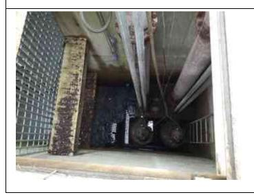
Inspect ID: 2022-0012 Title: 2604000003\_CELRC\_2022\_A\_0012\_1\_20220607T142146.jpg Rated Item: 7. Pumps Caption: Acceptable - PS-IW: Pumps not run due to low water in sump. Operator stated this low water is about as much water it receives. Pumps run very infrequently. No issues.
