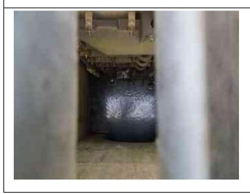
Inspect ID: 2022-0089 Title: 260400003\_CELRC\_2022\_A\_0089\_1\_20220609T144042.jpg Rated Item: 10. Sluice/ Slide Gates Caption: Acceptable - GN-3: Gate closed completely, sediment on bottom.
