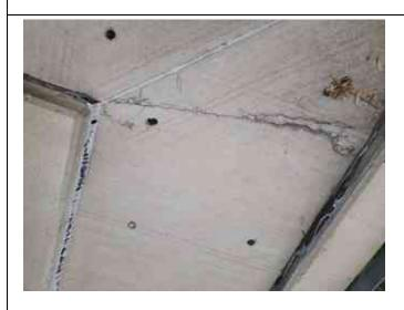
Inspect ID: 2022-0033 Title: 260400003\_CELRC\_2022\_A\_0033\_1\_20220607T151726.jpg Rated Item: 5. Plant Building Caption: Minimally Acceptable - PS-BR: Cracking in concrete.
