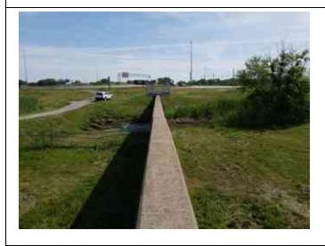
Inspect ID: 2022-0571 Title: 260400003\_CELRC\_2022\_A\_0571\_1\_20220610T143802.jpg Rated Item: 5. Tilting, Sliding or Settlement of Concrete Structures Caption: Minimally Acceptable - Floodwall is slightly tilted with 1 inch offset.
