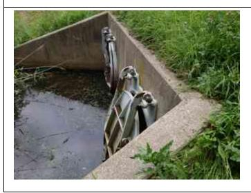
Inspect ID: 2022-0047 Title: 260400003\_CELRC\_2022\_A\_0047\_1\_20220607T171356.jpg Rated Item: 11. Flap Gates/ Flap Valves/ Pinch Valves Caption: Minimally Acceptable - GN-18: Flap gates are stuck open.
