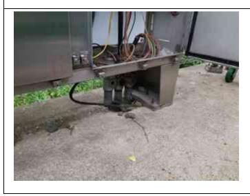
Inspect ID: 2022-0006 Title: 260400003\_CELRC\_2022\_A\_0006\_1\_20220607T141848.jpg Rated Item: 14. Electrical Systems Caption: Minimally Acceptable - PS-IW: Grounding conductor is frayed.
