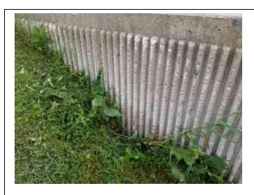
Inspect ID: 2022-0001 Title: 260400003\_CELRC\_2022\_A\_0001\_1\_20220607T133305.jpg Rated Item: 6. Foundation of Concrete Structures Caption: Minimally Acceptable - Depression along riverside of floodwall. 9 deep by 9x12.
