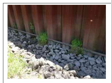
Inspect ID: 2022-0158 Title: 2604000003\_CELRC\_2022\_A\_0158\_1\_20220609T183951.jpg Rated Item: 9. Seepage Caption: Minimally Acceptable - Evidence of seepage at base by Colfax. Silt in some of the flanges at the landside base.
