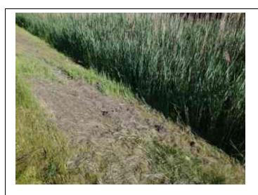
Inspect ID: 2022-0230 Title: 2604000003\_CELRC\_2022\_A\_0230\_1\_20220610T130801.jpg Rated Item: 2. Sod Cover Caption: Minimally Acceptable - Sod cover poor on landside slope.
