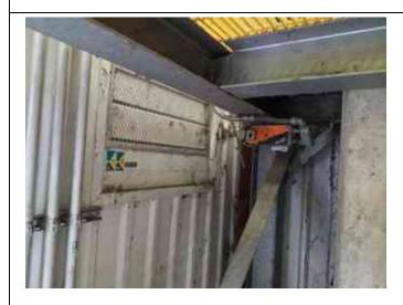
Inspect ID: 2022-0024 Title: 2604000003\_CELRC\_2022\_A\_0024\_1\_20220607T151235.jpg Rated Item: 5. Plant Building Caption: Minimally Acceptable - PS-BR: Louver actuator closes correctly when operated but has trouble opening.
