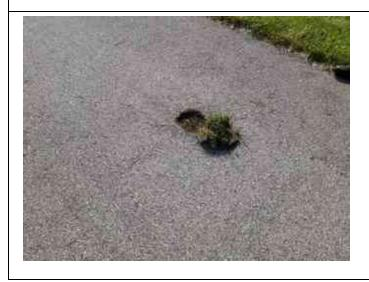
Inspect ID: 2022-0254 Title: 260400003\_CELRC\_2022\_A\_0254\_1\_20220610T132616.jpg Rated Item: 9. Cracking Caption: Minimally Acceptable - Crack in asphalt on crown
