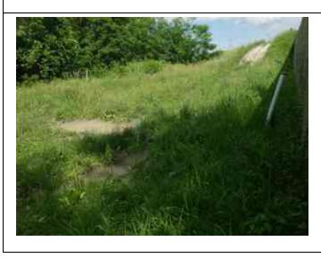
Inspect ID: 2022-0460 Title: 260400003\_CELRC\_2022\_A\_0460\_1\_20220609T192336.jpg Rated Item: 6. Foundation of Concrete Structures Caption: Minimally Acceptable - Pooling of water on landside base of floodwall.
