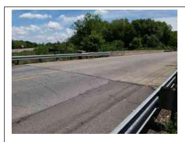
Inspect ID: 2022-0146 Title: 260400003\_CELRC\_2022\_A\_0146\_1\_20220609T183054.jpg Rated Item: 3. Closure Structures (Stop Log Closures and Gates) (A or U only) Caption: Acceptable - Guardrail blocking sandbag closure at Colfax.
