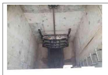
Inspect ID: 2022-0036 Title: 2604000015\_CELRC\_2022\_A\_0036\_1\_20220606T154006.jpg Rated Item: 10. Sluice/ Slide Gates Caption: Acceptable - 908: Gate closed completely.
