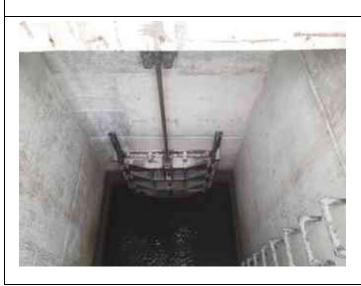
Inspect ID: 2022-0026 Title: 2604000015\_CELRC\_2022\_A\_0026\_1\_20220606T152524.jpg Rated Item: 10. Sluice/ Slide Gates Caption: Acceptable - 901: Gate closed completely. All gates were recently greased.
