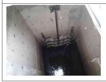
Inspect ID: 2022-0042 Title: 2604000015\_CELRC\_2022\_A\_0042\_1\_20220606T155312.jpg Rated Item: 10. Sluice/ Slide Gates Caption: Acceptable - 906: Gate closed completely.
