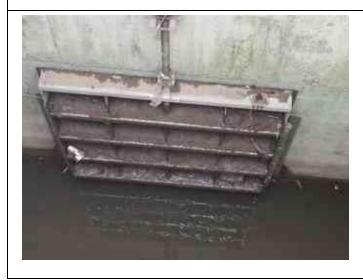
Inspect ID: 2022-0014 Title: 2604000009\_CELRC\_2022\_A\_0014\_5\_20220411T144245.jpg Rated Item: 10. Sluice/ Slide Gates Caption: Acceptable - MU-2: A little bit of silt.
