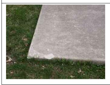
Inspect ID: 2022-0015 Title: 260400009\_CELRC\_2022\_A\_0015\_1\_20220411T132950.jpg Rated Item: 5. Plant Building Caption: Acceptable - PS-BA: Minor spalling on foundation pad.
