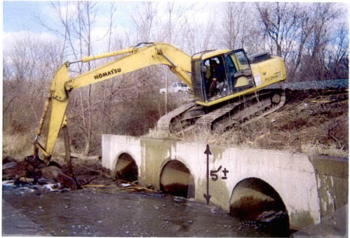
⑦ ADDITIONAL REMOVAL OF DEBRIS-NEXT DAY, (TOP OF ABUTMENT TO WATER LEVEL-APPROX. 5')
