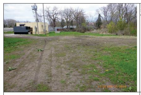
Inspect ID: LCMN\_2014\_a\_0064 Title: USACE\_CELRC\_LCMN\_2014\_a\_0064\_1.jpg Rated Item: 2. Sod Cover Caption: Rating: Minimally Acceptable; Remarks: Poor sod cover; Action: Seed
