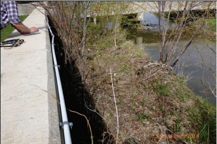
**Inspect ID:** LCMN\_2014\_a\_0016 **Title:** USACE\_CELRC\_LCMN\_2014\_a\_0016\_1.jpg **Rated Item:** 1. Unwanted Vegetation Growth **Caption:** Rating: Minimally Acceptable; Remarks: Trees on riverside of floodwall at Northcote; Action: Clear
