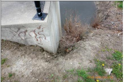
Inspect ID: LCMN\_2014\_a\_0063 Title: USACE\_CELRC\_LCMN\_2014\_a\_0063\_1.jpg Rated Item: 5. Concrete Surfaces (Such as gate wells, outfalls, intakes, or culverts) Caption: Rating: Minimally Acceptable; Remarks: Erosion next to outlet; Action: Fill
