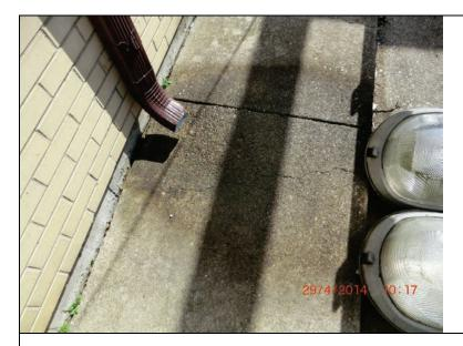
**Inspect ID:** LCMN\_2014\_a\_0087 **Title:** USACE\_CELRC\_LCMN\_2014\_a\_0087\_1.jpg **Rated Item:** 5. Plant Building **Caption:** Rating: Minimally Acceptable; Remarks: PSCAL: Exposed rebar; Action: Patch concrete
