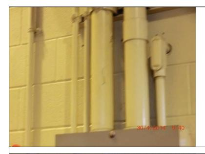
Inspect ID: LCMN\_2014\_a\_0083 Title: USACE\_CELRC\_LCMN\_2014\_a\_0083\_1.jpg Rated Item: 16. Enclosures, Panels, Conduit and Ducts Caption: Rating: Minimally Acceptable; Remarks: PS-OA: Paint peeling; Action: Repaint
