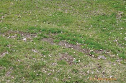
**Inspect ID:** LCMN\_2014\_a\_0054 **Title:** USACE\_CELRC\_LCMN\_2014\_a\_0054\_1.jpg **Rated Item:** 8. Depressions/ Rutting **Caption:** Rating: Acceptable; Remarks: Rutting on riverside slope; Action: Fill
