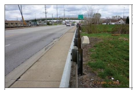
Inspect ID: LCMN\_2014\_a\_0040 Title: USACE\_CELRC\_LCMN\_2014\_a\_0040\_1.jpg Rated Item: 3. Closure Structures (Stop Log Closures and Gates) (A or U only) Caption: Rating: Acceptable; Remarks: Guardrail blocking closure wingwall; Action: Discuss alternatives and conduct a closure exercise at location to verify effectiveness of closure.
