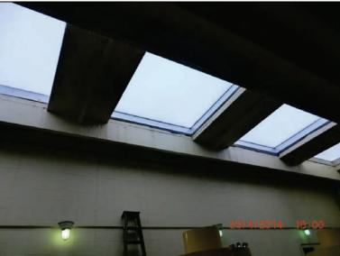
Inspect ID: LCMN\_2014\_a\_0086 Title: USACE\_CELRC\_LCMN\_2014\_a\_0086\_1.jpg Rated Item: 5. Plant Building Caption: Rating: Minimally Acceptable; Remarks: PSCAL: Broken concrete and leaking at skylights; Action: Seal cracks
