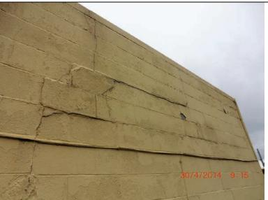
Inspect ID: LCMN\_2014\_a\_0098 Title: USACE\_CELRC\_LCMN\_2014\_a\_0098\_1.jpg Rated Item: 5. Plant Building Caption: Rating: Minimally Acceptable; Remarks: PS-HM: Cracking of masonry wall; Action: Seal
