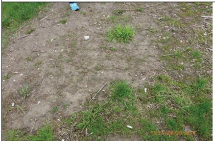
Inspect ID: LCMN\_2014\_a\_0065 Title: USACE\_CELRC\_LCMN\_2014\_a\_0065\_1.jpg Rated Item: 2. Sod Cover Caption: Rating: Minimally Acceptable; Remarks: Poor sod; Action: Seed
