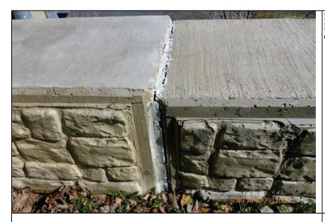
Inspect ID: LCMN\_2014\_a\_0015 Title: USACE\_CELRC\_LCMN\_2014\_a\_0015\_1.jpg Rated Item: 7. Monolith Joints Caption: Rating: Minimally Acceptable; Remarks: Joint cracked and requires caulking; Action: NA
