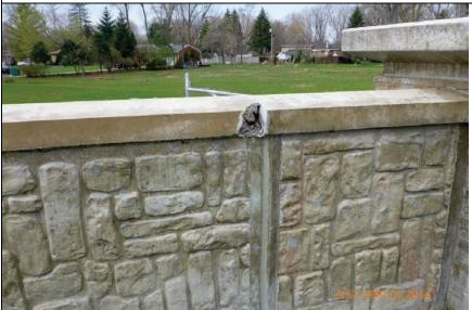
**Inspect ID:** LCMN\_2014\_a\_0017 **Title:** USACE\_CELRC\_LCMN\_2014\_a\_0017\_1.jpg **Rated Item:** 4. Concrete Surfaces **Caption:** Rating: Minimally Acceptable; Remarks: Concrete cap broken; Action: Patch
