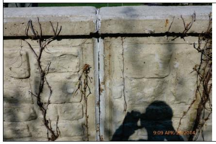
Inspect ID: LCMN\_2014\_a\_0001 Title: USACE\_CELRC\_LCMN\_2014\_a\_0001\_1.jpg Rated Item: 7. Monolith Joints Caption: Rating: Minimally Acceptable; Remarks: Monolith joint should be re-caulked on riverside; Action: Re-caulk
