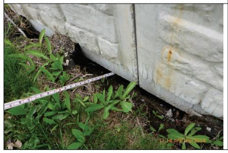
Inspect ID: LCMN\_2014\_a\_0036 Title: USACE\_CELRC\_LCMN\_2014\_a\_0036\_1.jpg Rated Item: 6. Foundation of Concrete Structures Caption: Rating: Minimally Acceptable; Remarks: 2 ft. deep settlement/erosion holes in fill material along base of floodwall.; Action: Fill with stone or grout
