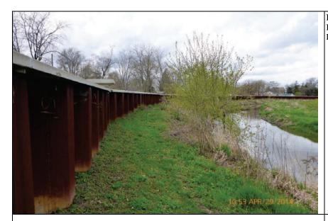
Inspect ID: LCMN\_2014\_a\_0023 Title: USACE\_CELRC\_LCMN\_2014\_a\_0023\_1.jpg Rated Item: 1. Unwanted Vegetation Growth Caption: Rating: Minimally Acceptable; Remarks: Tree on riverside of floodwall; Action: Clear
