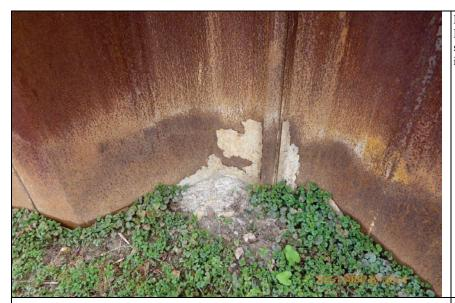
Inspect ID: LCMN\_2014\_a\_0066 Title: USACE\_CELRC\_LCMN\_2014\_a\_0066\_1.jpg Rated Item: 4. Concrete Surfaces Caption: Rating: Acceptable; Remarks: Steel sheetpile has minor corrosion at ground level, typical throughout; Action: Monitor for any increased scaling or section loss
