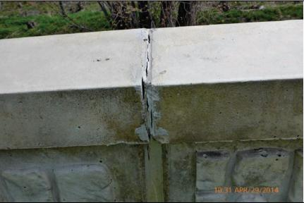
Inspect ID: LCMN\_2014\_a\_0019 Title: USACE\_CELRC\_LCMN\_2014\_a\_0019\_1.jpg Rated Item: 7. Monolith Joints Caption: Rating: Minimally Acceptable; Remarks: Joint deterioration; Action: Re-caulk
