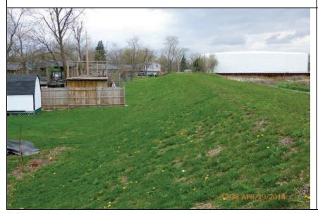
Inspect ID: LCMN\_2014\_a\_0049 Title: USACE\_CELRC\_LCMN\_2014\_a\_0049\_1.jpg Rated Item: 3. Encroachments Caption: Rating: Minimally Acceptable; Remarks: Fence near landside toe; Action: Remove within 15 ft of the levee or request permit
