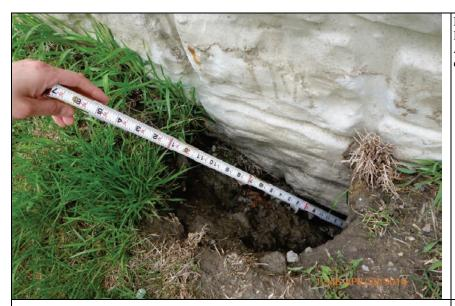
Inspect ID: LCMN\_2014\_a\_0045 Title: USACE\_CELRC\_LCMN\_2014\_a\_0045\_1.jpg Rated Item: 6. Foundation of Concrete Structures Caption: Rating: Minimally Acceptable; Remarks: 2 ft. deep large settlement/erosion holes in fill material along base of floodwall.; Action: Fill with stone or grout
