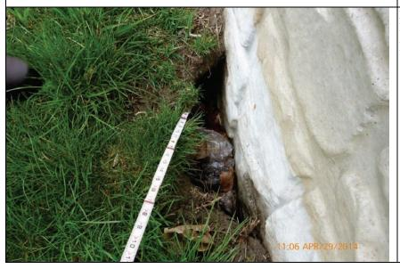
Inspect ID: LCMN\_2014\_a\_0031 Title: USACE\_CELRC\_LCMN\_2014\_a\_0031\_1.jpg Rated Item: 6. Foundation of Concrete Structures Caption: Rating: Minimally Acceptable; Remarks: 3 ft. deep settlement/erosion holes in fill material along base of floodwall.; Action: Fill with stone or grout
