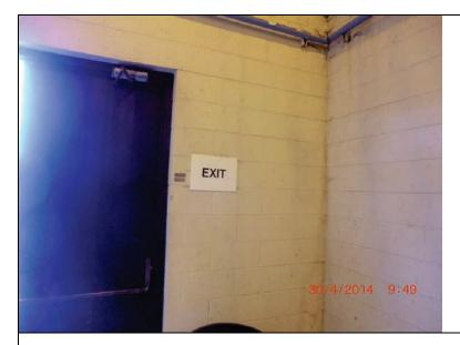
Inspect ID: LCMN\_2014\_a\_0075 Title: USACE\_CELRC\_LCMN\_2014\_a\_0075\_1.jpg Rated Item: 3. Safety Compliance Caption: Rating: Minimally Acceptable; Remarks: PS-OA: Non-standard exit sign; Action: Replace with compliant signage
