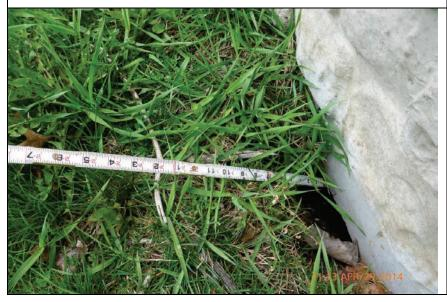
Inspect ID: LCMN\_2014\_a\_0034 Title: USACE\_CELRC\_LCMN\_2014\_a\_0034\_1.jpg Rated Item: 6. Foundation of Concrete Structures Caption: Rating: Minimally Acceptable; Remarks: 1.5 ft. deep settlement/erosion holes in fill material along base of floodwall.; Action: Fill with stone or grout
