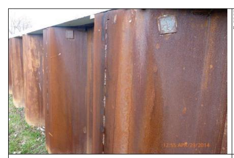
Inspect ID: LCMN\_2014\_a\_0057 Title: USACE\_CELRC\_LCMN\_2014\_a\_0057\_1.jpg Rated Item: 4. Concrete Surfaces Caption: Rating: Acceptable; Remarks: It is not normal practice or recommended to weld the interlocks of the sheet pile; Action: Monitor
