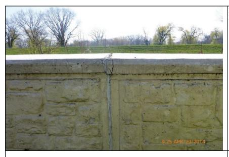
Inspect ID: LCMN\_2014\_a\_0007 Title: USACE\_CELRC\_LCMN\_2014\_a\_0007\_1.jpg Rated Item: 7. Monolith Joints Caption: Rating: Minimally Acceptable; Remarks: Joint sealant deteriorating; Action: Re-caulk
