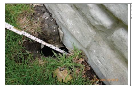
Inspect ID: LCMN\_2014\_a\_0028 Title: USACE\_CELRC\_LCMN\_2014\_a\_0028\_1.jpg Rated Item: 6. Foundation of Concrete Structures Caption: Rating: Minimally Acceptable; Remarks: 3 ft. deep settlement/erosion holes in fill material along base of floodwall.; Action: Fill with stone or grout
