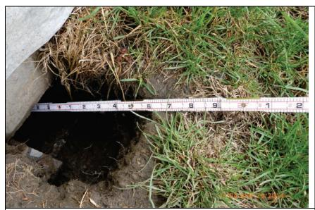
**Inspect ID:** LCMN\_2014\_a\_0030 **Title:** USACE\_CELRC\_LCMN\_2014\_a\_0030\_1.jpg **Rated Item:** 6. Foundation of Concrete Structures **Caption:** Rating: Minimally Acceptable; Remarks: 1.5 ft. deep settlement/erosion holes in fill material along base of floodwall.; Action: Fill with stone or grout
