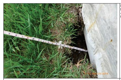
Inspect ID: LCMN\_2014\_a\_0035 Title: USACE\_CELRC\_LCMN\_2014\_a\_0035\_1.jpg Rated Item: 6. Foundation of Concrete Structures Caption: Rating: Minimally Acceptable; Remarks: 2 ft. deep settlement/erosion holes in fill material along base of floodwall.; Action: Fill with stone or grout
