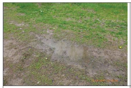
Inspect ID: LCMN\_2014\_a\_0061 Title: USACE\_CELRC\_LCMN\_2014\_a\_0061\_1.jpg Rated Item: 8. Depressions/ Rutting Caption: Rating: Minimally Acceptable; Remarks: Rut on riverside with ponded water; Action: Fill
