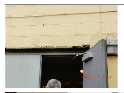
Inspect ID: LCMN\_2014\_a\_0095 Title: USACE\_CELRC\_LCMN\_2014\_a\_0095\_1.jpg Rated Item: 5. Plant Building Caption: Rating: Minimally Acceptable; Remarks: PS-HM: Deteriorating lintel; Action: Fix
