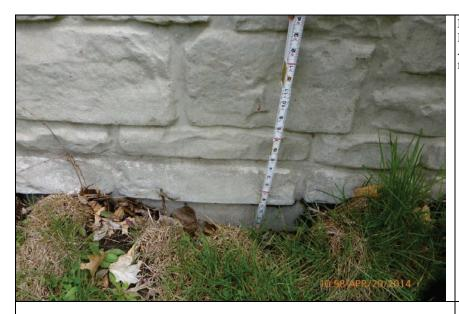
Inspect ID: LCMN\_2014\_a\_0026 Title: USACE\_CELRC\_LCMN\_2014\_a\_0026\_1.jpg Rated Item: 6. Foundation of Concrete Structures Caption: Rating: Minimally Acceptable; Remarks: 1 ft. deep settlement/erosion holes in fill material along base of floodwall.; Action: Fill with stone or grout
