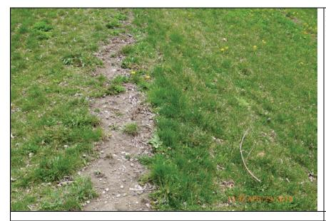
Inspect ID: LCMN\_2014\_a\_0047 Title: USACE\_CELRC\_LCMN\_2014\_a\_0047\_1.jpg Rated Item: 8. Depressions/ Rutting Caption: Rating: Acceptable; Remarks: Rutting on landside slope; Action: Fill
