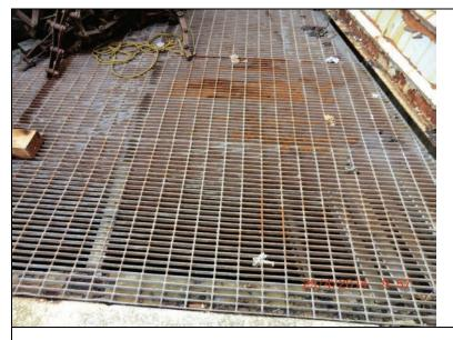
Inspect ID: LCMN\_2014\_a\_0093 Title: USACE\_CELRC\_LCMN\_2014\_a\_0093\_1.jpg Rated Item: 21. Other Metallic Items (Equipment, Ladders, Platform Anchors, etc) Caption: Rating: Minimally Acceptable; Remarks: PS-CAL: Rusted grate; Action: Clean and repaint
