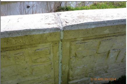
**Inspect ID:** LCMN\_2014\_a\_0004 **Title:** USACE\_CELRC\_LCMN\_2014\_a\_0004\_1.jpg **Rated Item:** 7. Monolith Joints **Caption:** Rating: Minimally Acceptable; Remarks: Joint sealant deterioration on landside, prior issue still exists in 2014; Action: Re-caulk
