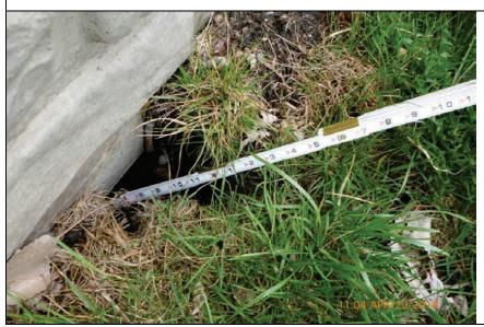
Inspect ID: LCMN\_2014\_a\_0029 Title: USACE\_CELRC\_LCMN\_2014\_a\_0029\_1.jpg Rated Item: 6. Foundation of Concrete Structures Caption: Rating: Minimally Acceptable; Remarks: 3 ft. deep settlement/erosion holes in fill material along base of floodwall, on landside.; Action: Fill with stone or grout
