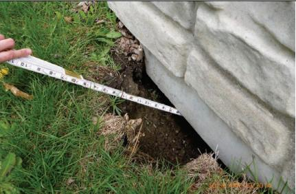
Inspect ID: LCMN\_2014\_a\_0027 Title: USACE\_CELRC\_LCMN\_2014\_a\_0027\_1.jpg Rated Item: 6. Foundation of Concrete Structures Caption: Rating: Minimally Acceptable; Remarks: 2 ft. deep settlement/erosion holes in fill material along base of floodwall.; Action: Fill with stone or grout
