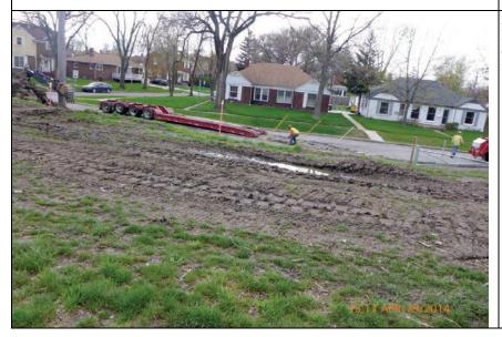
Inspect ID: LCMN\_2014\_a\_0062 Title: USACE\_CELRC\_LCMN\_2014\_a\_0062\_1.jpg Rated Item: 2. Sod Cover Caption: Rating: Minimally Acceptable; Remarks: Rutting due to temporary construction; Action: Check that the levee is restored once construction is complete
