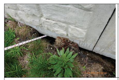
Inspect ID: LCMN\_2014\_a\_0037 Title: USACE\_CELRC\_LCMN\_2014\_a\_0037\_1.jpg Rated Item: 6. Foundation of Concrete Structures Caption: Rating: Minimally Acceptable; Remarks: 2 ft. deep settlement/erosion holes in fill material along base of floodwall.; Action: Fill with stone or grout
