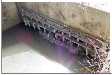
Inspect ID: LCMN\_2014\_a\_0069 Title: USACE\_CELRC\_LCMN\_2014\_a\_0069\_1.jpg Rated Item: 1. Vegetation and Obstructions Caption: Rating: Minimally Acceptable; Remarks: MU-2: Outlet clogged with trash and silt; Action: Clean
