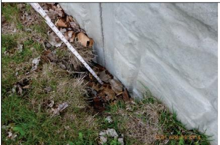
Inspect ID: LCMN\_2014\_a\_0058 Title: USACE\_CELRC\_LCMN\_2014\_a\_0058\_1.jpg Rated Item: 6. Foundation of Concrete Structures Caption: Rating: Minimally Acceptable; Remarks: 1 ft. deep settlement/erosion holes in fill material along base of floodwall.; Action: Fill with stone or grout
