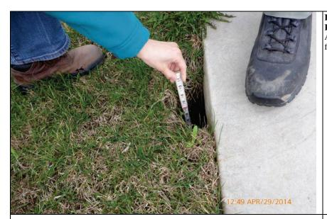
Inspect ID: LCMN\_2014\_a\_0053 Title: USACE\_CELRC\_LCMN\_2014\_a\_0053\_1.jpg Rated Item: 6. Foundation of Concrete Structures Caption: Rating: Minimally Acceptable; Remarks: Deep settlement/erosion hole in fill material along base of floodwall.; Action: Fill with stone or grout
