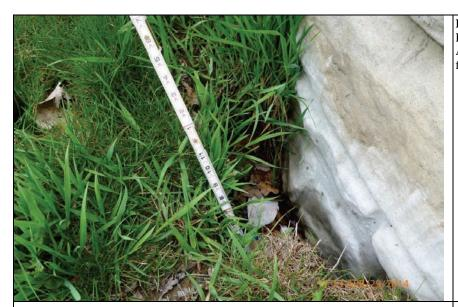
Inspect ID: LCMN\_2014\_a\_0032 Title: USACE\_CELRC\_LCMN\_2014\_a\_0032\_1.jpg Rated Item: 6. Foundation of Concrete Structures Caption: Rating: Minimally Acceptable; Remarks: 3 ft. deep settlement/erosion holes in fill material along base of floodwall, on landside.; Action: Fill with stone or grout
