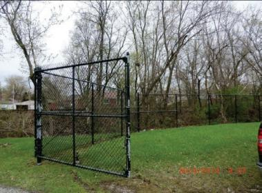
Inspect ID: LCMN\_2014\_a\_0078 Title: USACE\_CELRC\_LCMN\_2014\_a\_0078\_1.jpg Rated Item: 6. Fencing and Gates Caption: Rating: Minimally Acceptable; Remarks: PS-OA: Damaged fence; Action: Repair
