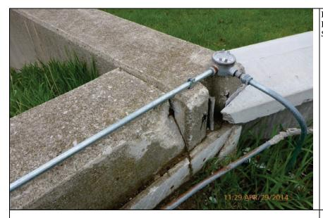
Inspect ID: LCMN\_2014\_a\_0039 Title: USACE\_CELRC\_LCMN\_2014\_a\_0039\_1.jpg Rated Item: 4. Concrete Surfaces Caption: Rating: Minimally Acceptable; Remarks: Spalling and exposed rebar; Action: Clean rebar and patch concrete
