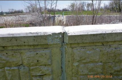
**Inspect ID:** LCMN\_2014\_a\_0008 **Title:** USACE\_CELRC\_LCMN\_2014\_a\_0008\_1.jpg **Rated Item:** 7. Monolith Joints **Caption:** Rating: Minimally Acceptable; Remarks: Joint sealant deteriorating; Action: Re-caulk
