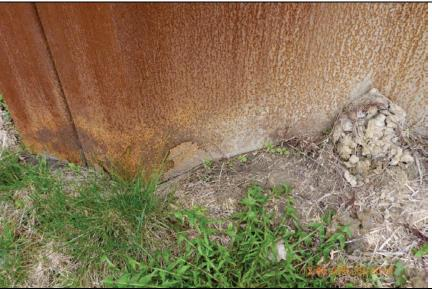
Inspect ID: LCMN\_2014\_a\_0052 Title: USACE\_CELRC\_LCMN\_2014\_a\_0052\_1.jpg Rated Item: 4. Concrete Surfaces Caption: Rating: Acceptable; Remarks: Scaling at base of sheetpile; Action: Monitor for any increased scaling or section loss; and possible sheetpile alignment issues
