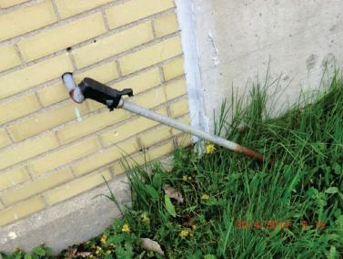
Inspect ID: LCMN\_2014\_a\_0100 Title: USACE\_CELRC\_LCMN\_2014\_a\_0100\_1.jpg Rated Item: 16. Enclosures, Panels, Conduit and Ducts Caption: Rating: Minimally Acceptable; Remarks: PS-HM: Corroded conduit exiting the wall and laying on the ground; Action: Repair
