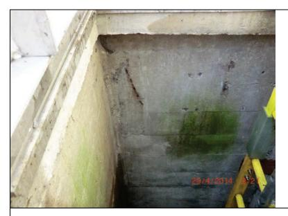
**Inspect ID:** LCMN\_2014\_a\_0084 **Title:** USACE\_CELRC\_LCMN\_2014\_a\_0084\_1.jpg **Rated Item:** 5. Plant Building **Caption:** Rating: Minimally Acceptable; Remarks: PS-BA: Exposed rebar in concrete; Action: Patch
