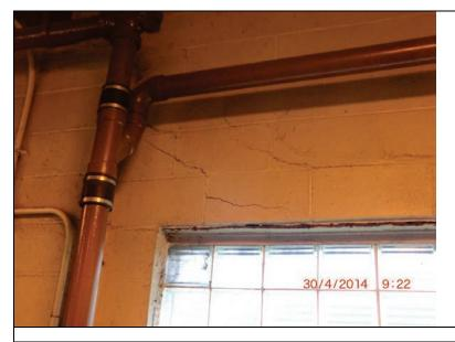
Inspect ID: LCMN\_2014\_a\_0099 Title: USACE\_CELRC\_LCMN\_2014\_a\_0099\_1.jpg Rated Item: 5. Plant Building Caption: Rating: Minimally Acceptable; Remarks: PS-HM: Cracking of masonry wall; Action: Seal
