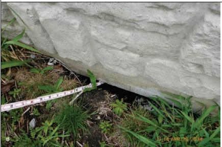
Inspect ID: LCMN\_2014\_a\_0038 Title: USACE\_CELRC\_LCMN\_2014\_a\_0038\_1.jpg Rated Item: 6. Foundation of Concrete Structures Caption: Rating: Minimally Acceptable; Remarks: 1 ft. deep settlement/erosion holes in fill material along base of floodwall.; Action: Fill with stone or grout
