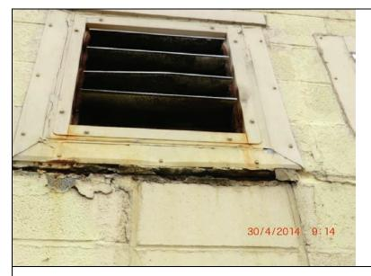
Inspect ID: LCMN\_2014\_a\_0097 Title: USACE\_CELRC\_LCMN\_2014\_a\_0097\_1.jpg Rated Item: 5. Plant Building Caption: Rating: Minimally Acceptable; Remarks: PS-HM: Masonry under vent deteriorating; Action: Repair
