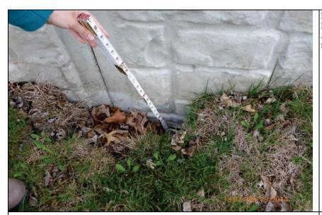
Inspect ID: LCMN\_2014\_a\_0059 Title: USACE\_CELRC\_LCMN\_2014\_a\_0059\_1.jpg Rated Item: 6. Foundation of Concrete Structures Caption: Rating: Minimally Acceptable; Remarks: 1.5 ft. deep settlement/erosion holes in fill material along base of floodwall.; Action: Fill with stone
