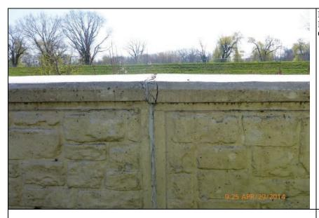
Inspect ID: LCMN\_2014\_a\_0009 Title: USACE\_CELRC\_LCMN\_2014\_a\_0009\_1.jpg Rated Item: 4. Concrete Surfaces Caption: Rating: Minimally Acceptable; Remarks: Cracks in concrete cap and spalling; Action: Patch
