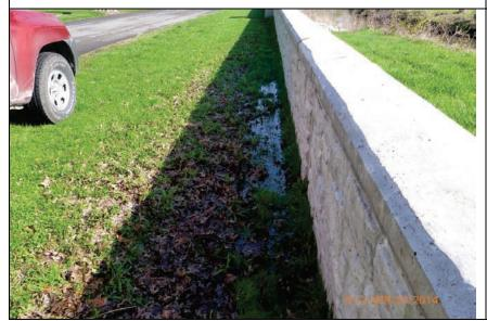
Inspect ID: LCMN\_2014\_a\_0006 Title: USACE\_CELRC\_LCMN\_2014\_a\_0006\_1.jpg Rated Item: 6. Foundation of Concrete Structures Caption: Rating: Minimally Acceptable; Remarks: Water ponding on landside floodwall; Action: Grade to drain away from wall
