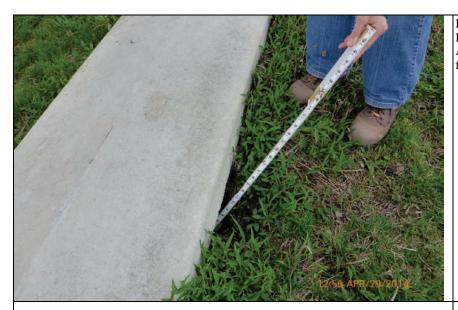
**Inspect ID:** LCMN\_2014\_a\_0056 **Title:** USACE\_CELRC\_LCMN\_2014\_a\_0056\_1.jpg **Rated Item:** 6. Foundation of Concrete Structures **Caption:** Rating: Minimally Acceptable; Remarks: 1 ft. deep settlement/erosion holes in fill material along base of floodwall.; Action: Fill with stone or grout
