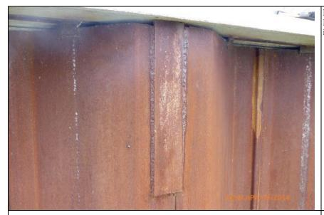
Inspect ID: LCMN\_2014\_a\_0024 Title: USACE\_CELRC\_LCMN\_2014\_a\_0024\_1.jpg Rated Item: 4. Concrete Surfaces Caption: Rating: Acceptable; Remarks: Sheetpile interlock joint needs repairing.; Action: monitor the existing splice repair
