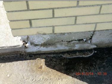
Inspect ID: LCMN\_2014\_a\_0088 Title: USACE\_CELRC\_LCMN\_2014\_a\_0088\_1.jpg Rated Item: 5. Plant Building Caption: Rating: Minimally Acceptable; Remarks: PSCAL: Spalling in foundation slab; Action: Patch
