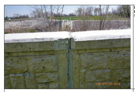
Inspect ID: LCMN\_2014\_a\_0013 Title: USACE\_CELRC\_LCMN\_2014\_a\_0013\_1.jpg Rated Item: 4. Concrete Surfaces Caption: Rating: Minimally Acceptable; Remarks: Spalling on landside floodwall; Action: Patch
