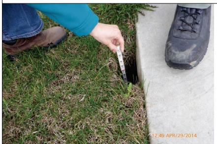
Inspect ID: LCMN\_2014\_a\_0051 Title: USACE\_CELRC\_LCMN\_2014\_a\_0051\_1.jpg Rated Item: 6. Foundation of Concrete Structures Caption: Rating: Minimally Acceptable; Remarks: 6 ft. deep settlement/erosion holes in fill material along base of floodwall.; Action: Fill with stone or grout
