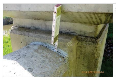
Inspect ID: LCMN\_2014\_a\_0002 Title: USACE\_CELRC\_LCMN\_2014\_a\_0002\_1.jpg Rated Item: 7. Monolith Joints Caption: Rating: Minimally Acceptable; Remarks: Joint sealant deterioration; Action: Re-caulk
