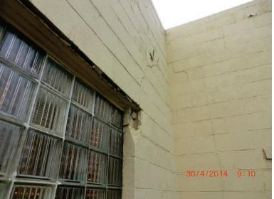
Inspect ID: LCMN\_2014\_a\_0096 Title: USACE\_CELRC\_LCMN\_2014\_a\_0096\_1.jpg Rated Item: 5. Plant Building Caption: Rating: Minimally Acceptable; Remarks: PS-HM: Broken masonry at south window; Action: Fix masonry
